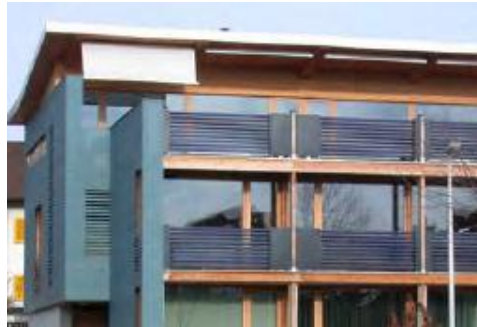
Fig. 2: Evacuated tube collector used as plate used
