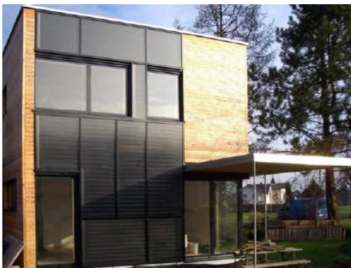
Fig. 3: Façade integration of glazed plate collector
