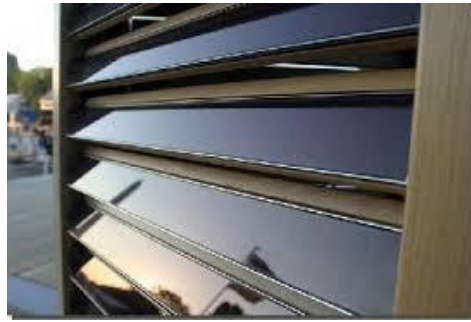
Fig. 15: PV shade Screens
