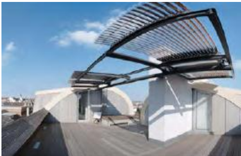
Fig. 1: Evacuated tube collector used as desk sun shading
