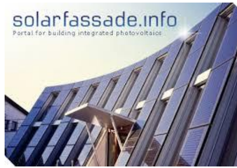
Fig. 12: PV adapted for the entrance foyer
