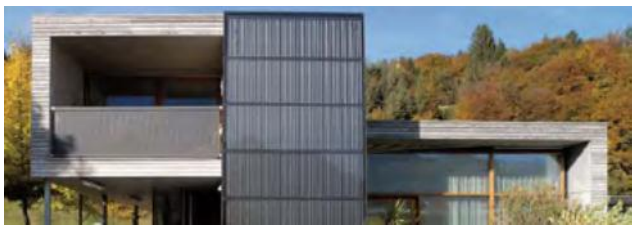
Fig. 6: Façade integrated with glazed PV collectors
