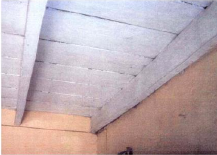
Plate 2. Use of well-seasoned hard wood as a floor slab in a vernacular building in Akure, Nigeria. Retrieved from Prucnal – Ogunsote (n.d.).
